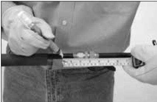
3. Heat shrink sleeves are 5 in. (125 mm) long. Mark the tube to center the sleeve over the fitting. The sleeve should overlap the jacket on the tube by a minimum of 1 in. (25 mm).
