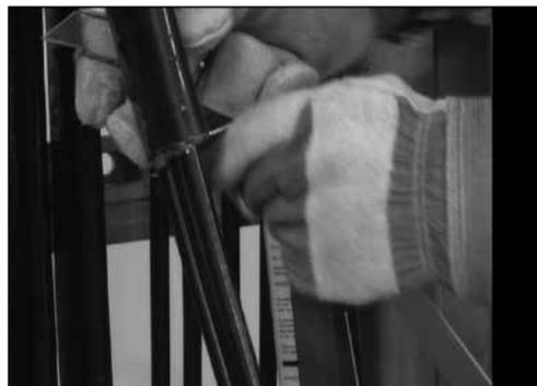
5. Score the aluminum stiffening plate with a knife and break off or cut with tin snips to remove.
