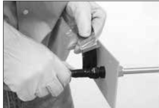
4. When applying the tape, keep the backing in place as long as possible. If the tape comes in contact with itself it will bond immediately.
