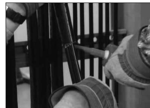
6. Apply silicone sealant to the cut seam where the outer jacket was removed.
