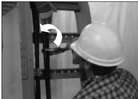
2. Make the bend with the flat side of the multijacketed tubing bundle following the radius of the tubing tray.
