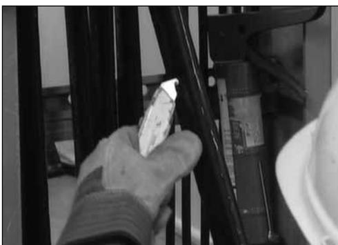
2. Slice outer jacket axially and remove.
