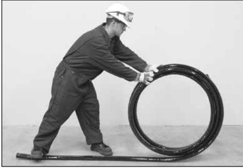
**Method 2:** Use a second smaller spool to straighten the product as it is taken off of the larger shipping spool.
