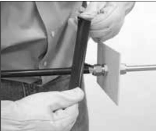
1. For the first layer, use a length of 8 to 10 in. (200 to 250 mm). **DO NOT REMOVE THE BACKING LAYER!**
