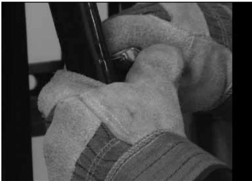
1. Cut outer jacket of multijacketed tubing to desired length. Do not cut into the tubing jacket on the individual tubes.
