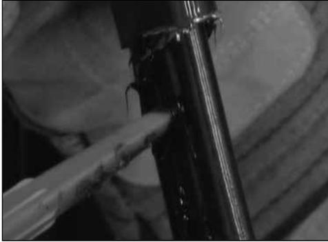
7. Apply silicone sealant between individual tubes, on both sides, to ensure a good seal is created.
