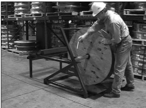
2. Use ramp to load spool and fit spindle into C-bracket on stand. Install safety pins through holes in C-bracket to secure spool in stand.
