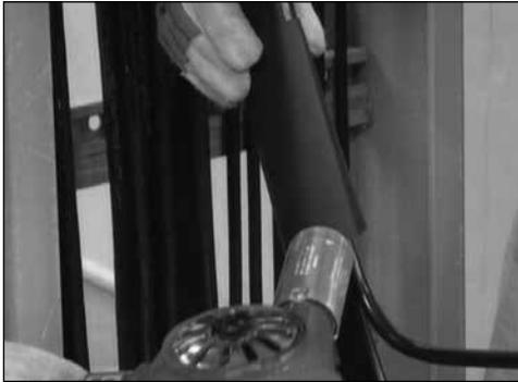
8. Center the heat shrink sleeve over the cut seam where outer jacket was removed.
