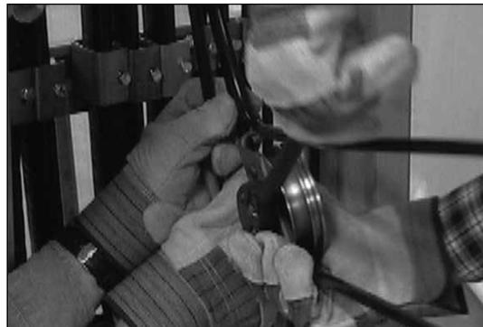
2. Use groove in bending shoe which best fits the tubing. Holding tubing securely, use 1/2 in. square drive ratchet to rotate shoe and bend tubing to desired angle.
