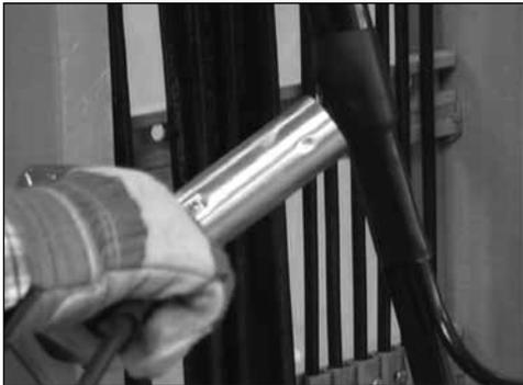
9. Use a heat gun to shrink the sleeve over the tubing. Move the heat source back and forth over the sleeve applying heat evenly.
